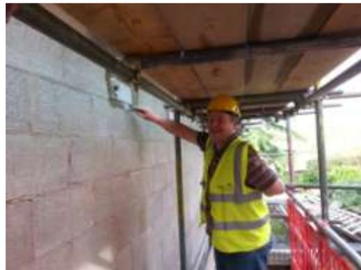
Above, the Schwegler Lightweight Swift Box 1A designed for fitting into plastered and insulated walls. W 340mm x H 135mm x D 150mm (plus 17mm for the protruding entrance ring)
