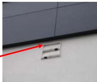
Schwegler make several designs of Swift nest box that can be sunk into the walls of brick or block built buildings, or bolted on to the surface.
